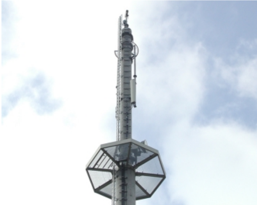
Illustration 5 FIRE-WATCH camera unit mounted on a radio antenna
