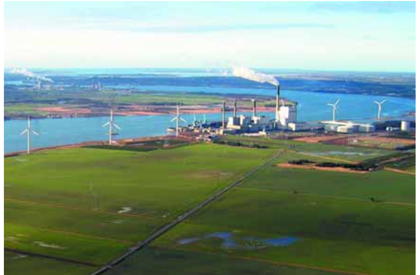
Technologies continue to be developed to improve the environmental performance of coal fired power stations – the Nordjyllandsværket coal fired power station in Denmark has an efficiency level of 47%. Photograph courtesy of Elsam. Photographer Gert Jensen.
