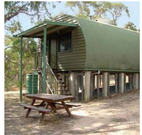
Mack Creek Hut, Para Wirra Conservation Park
