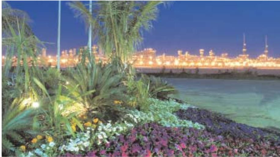
The Haradh-3 natural gas processing plant southwest of Dhahran
