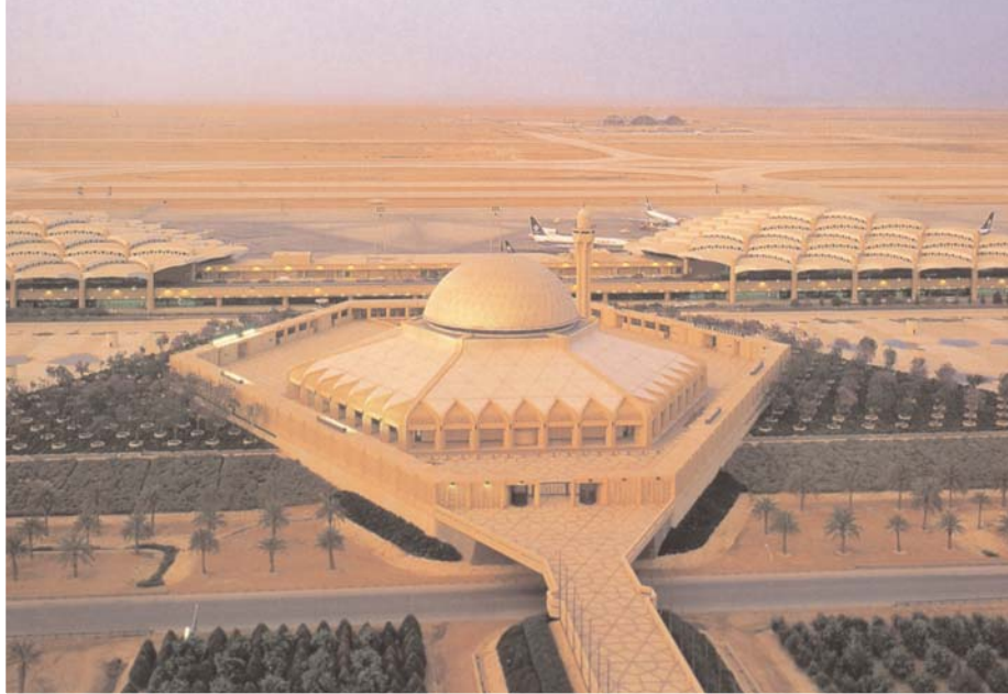
King Khalid International Airport in Riyadh
