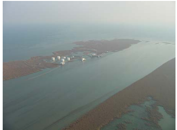
Figure 10. Overview for North Pass spills looking NE along North Pass (9/25/04).
