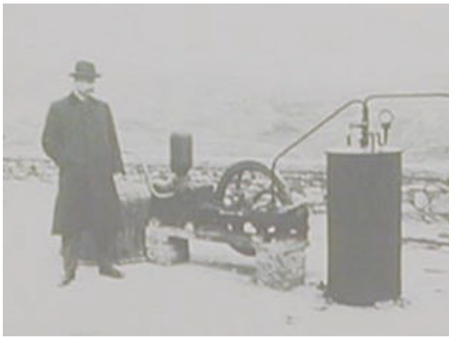
Figure 3. Prince Ginori Conti and the 10-kW experimental power plant, Larderello, Italy, 1994 (courtesy of ENEL).
