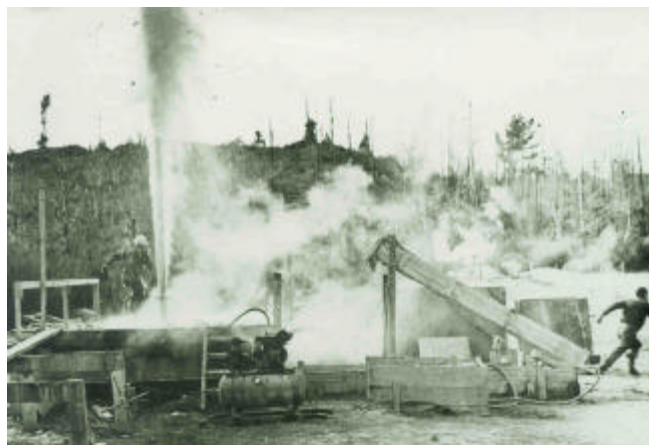
Figure 8. Drilling a Wairakei, New Zealand, 1950s (courtesy of Ian Thain).
