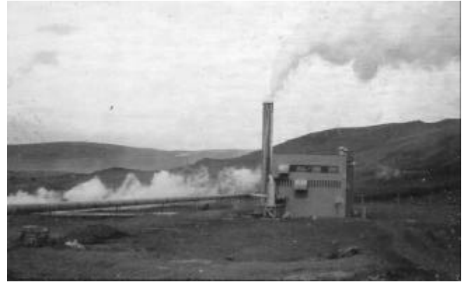
Figure 15. First geothermal plant in Iceland at Namafjall, 1969, 3-MW non-condensing plant.
