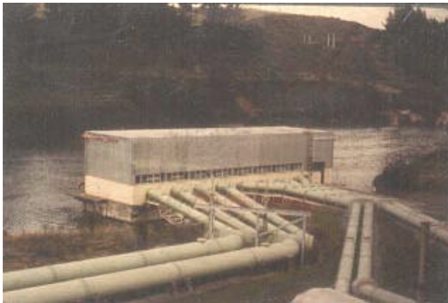
Figure 10. Wairakei power plant with Waikato River in background, New Zealand.
