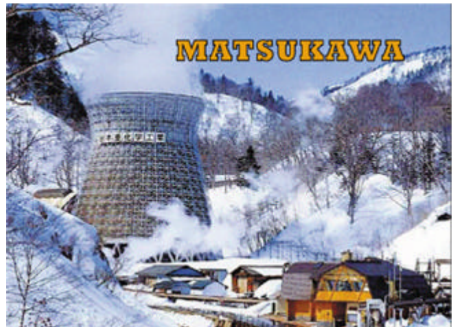
Figure 13. First power plant in Japan, 23-MW “dry steam” at Matsukawa.
