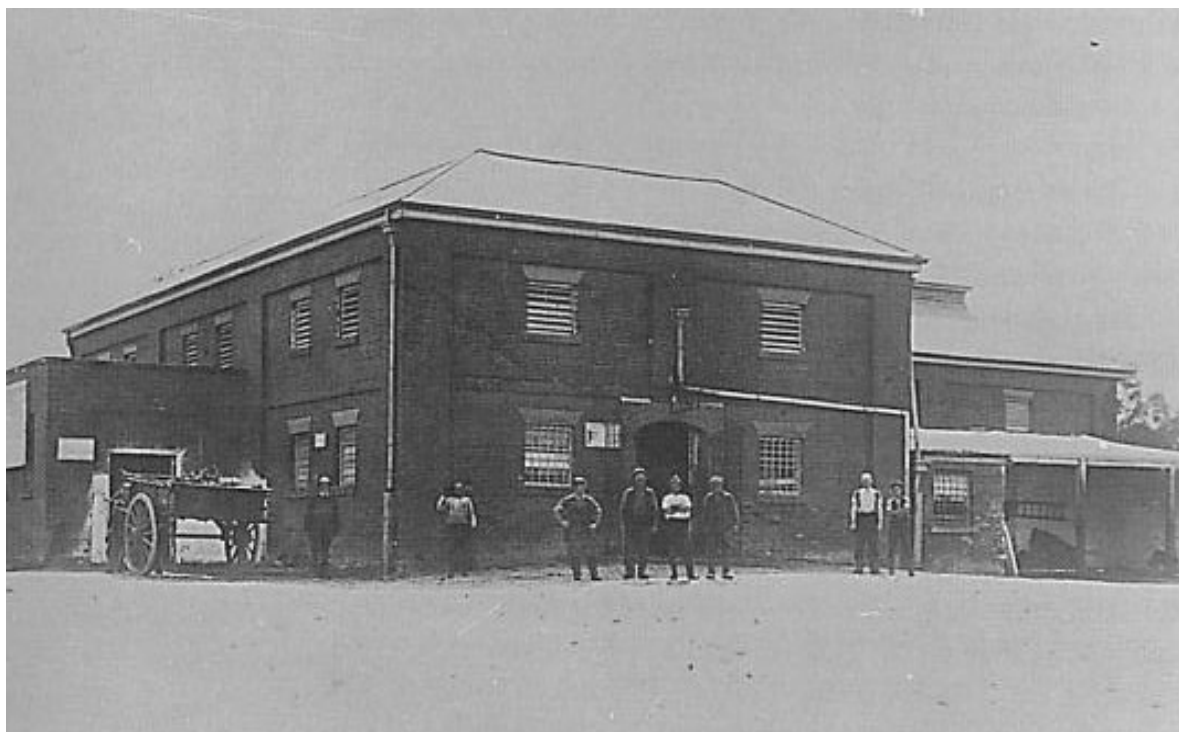
Figures Two images of the Council's Slaughterhouse in Park 27. To the left, an exterior photograph of the two storey brick structure c.1914 with galvanised iron roof with annex structures to left and right. This image, having regard to extant maps, appears to be looking north at the structure. Source: MLSA B267; Morton 1996, p. 156. To the right, an interior photograph c.1910 of the Slaughterhouse with its timber posts and beams. Source: MLSA B268; Morton 1996, p. 127.
