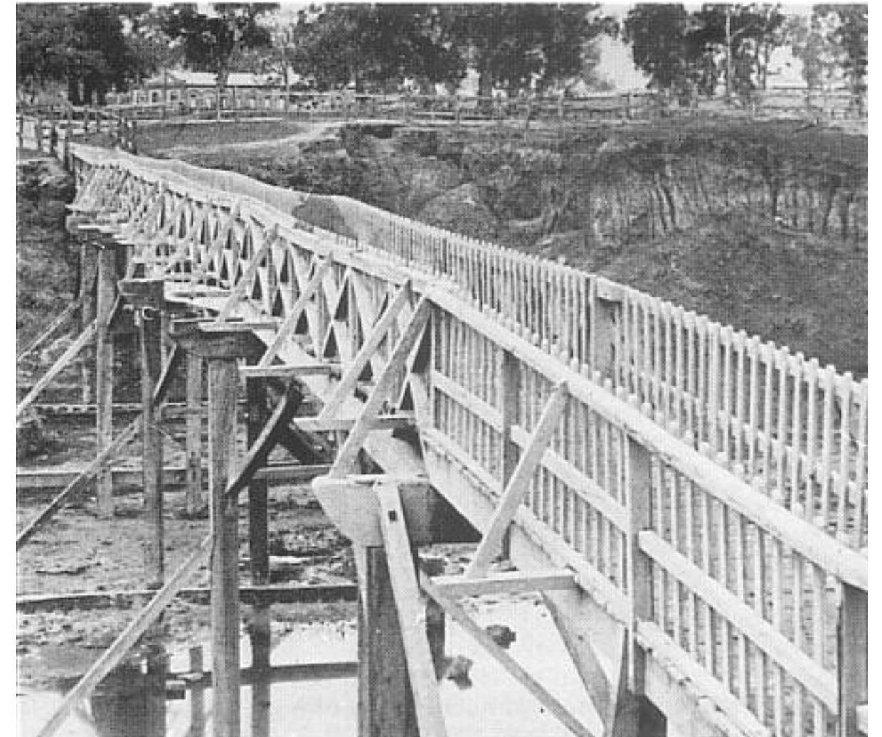
Figure Photograph of the timber "Frome Foot Bridge" over the River Torrens that existed from c.1863 to 1869. Note the timber Exhibition Building to the rear of the photograph together with the mature Eucalyptus spp along Frome Road and Victoria Drive alignment, and the extensive use of timber post and double rail fencing at the rear and along roadways. Source: MLSA B3324; Marsden et al 1990.
