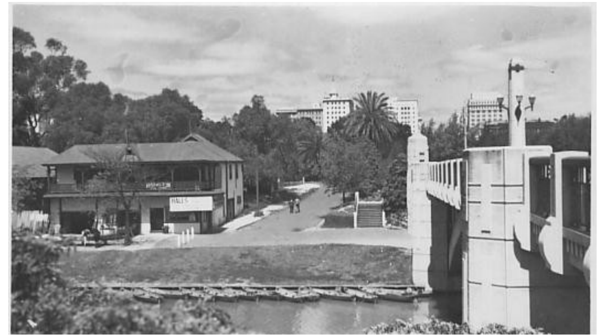
Figure Rose series P9499 black and white postcard of the side of Adelaide Bridge and Jolley's Boathouse in c.1930. Note the extensive form of the Boathouse, and the extant staircase and plantings behind, and the since removed palm tree. Source: private collection.
