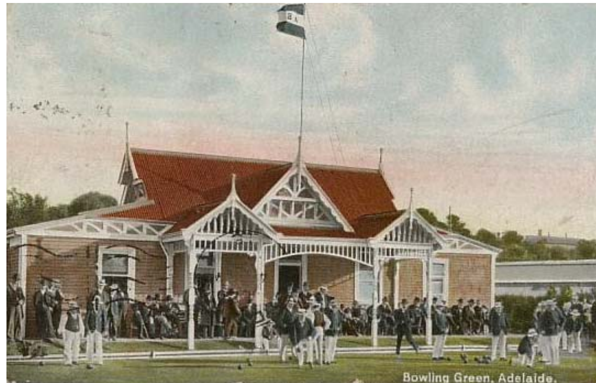
Figure The Adelaide Bowling Club “temporary club house” in c.1900 as depicted in a watercolour postcard. While ‘temporary’ it was clearly a fashionable Federation style timber fretwork design with finials and gables. Image is looking south-south-west along the Kintore Avenue alignment. Source: private collection.
