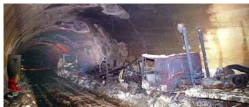
Figure 2. Aftermath of the 1999 Mont Blanc tunnel fire.
