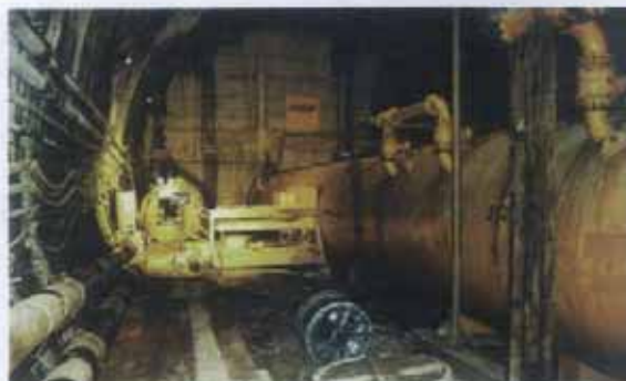
Above: Compressed air-lock in use in the Siegaue tunnel
