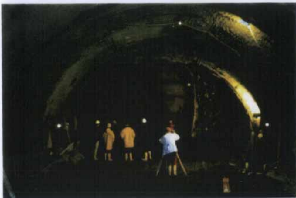
Left: Roof beam method being used in the Schulwald tunnel
