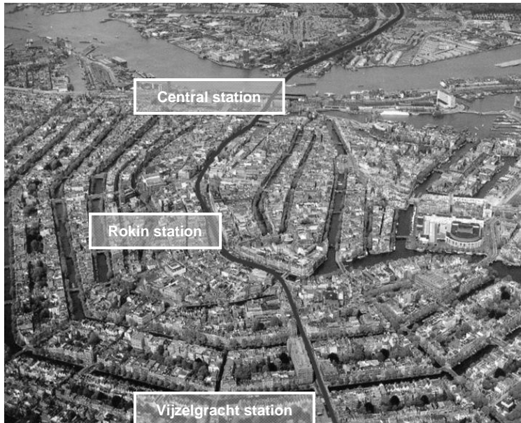
Fig. 1: Aerial view of the North-South Line in Amsterdam.
