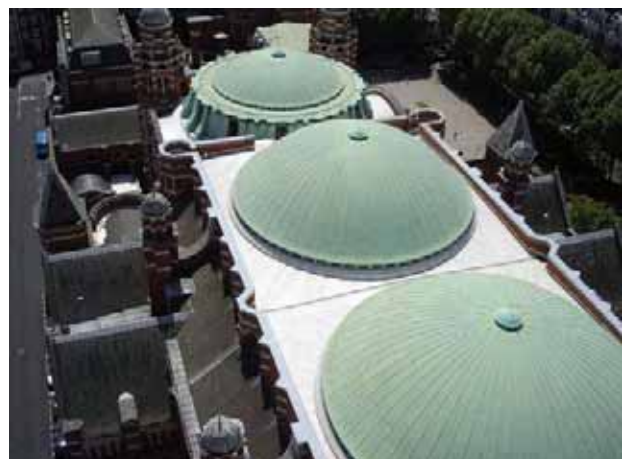
Figure 16: Aerial photo, Cathedral Roof
