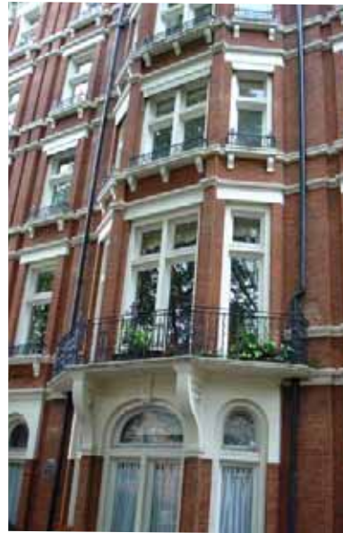
Figure 37: Bay windows. Nos 1-24 Morpeth Mansions
