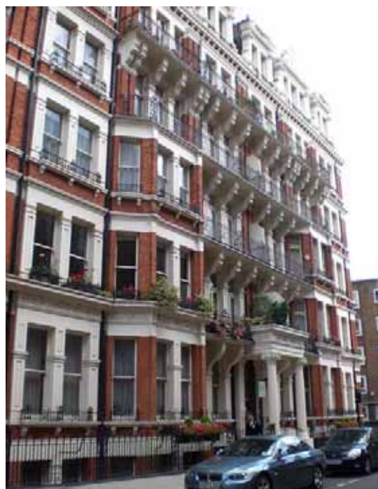
Figure 34: Cardinal Mansions, Carlisle Place
