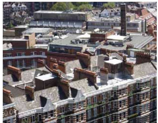
Figure 66: Ashley Garden Thirleby Road roofprofile showing pitched roofs with stout brick chimneys. Plant housings and lift overruns are incongruous features on the roofscape.
