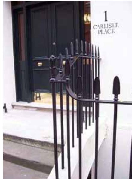
Figure 75: Replica cast iron Spearhead railings at No.1 Carlisle Place
