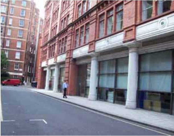
Figure 74: Loading bays on Greencoat Row
