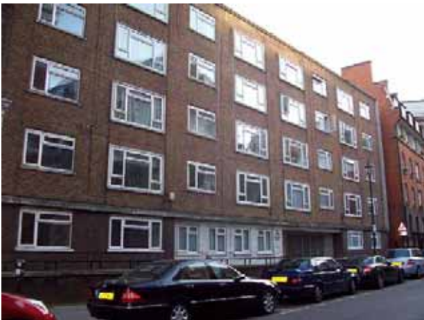
Figure 104: Victoria House, Francis Street
