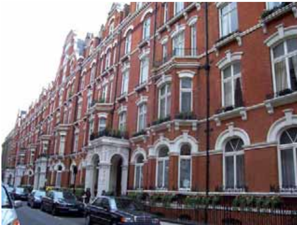
Figure 27: No. 41-85 Carlisle Mansions, western facade of Carlisle Place
