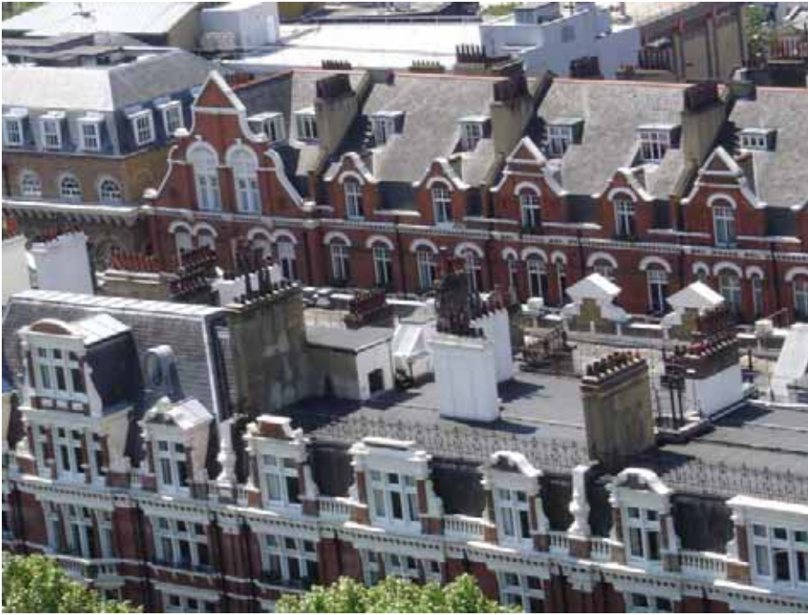
Figure 65: Roof profile showing Dutch gables of Carlisle Place (background) and grand mansard on Morpeth Terrace (foreground)
