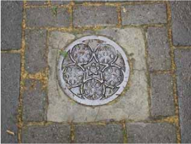
Figure 95: Coal Hole Cover. Morpeth Terrace
