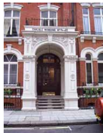
Figures 30, 31 & 32: Carlisle Mansion Porches (left to right) Nos. 21-35, Nos. 1-20 and Nos. 41-85
