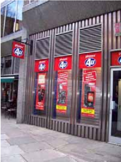
Figure 102: Brash signage on Ashdown House rear elevation
