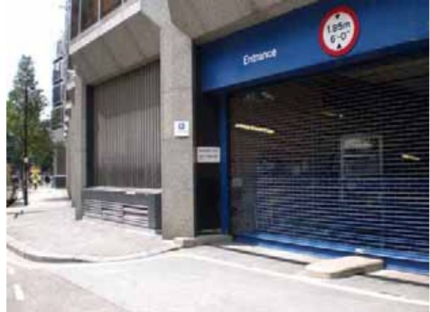
Figure 100: Service entrances on Howick Place
