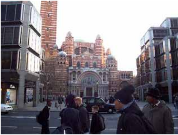
Figure 64: Cathedral viewed from Victoria Street through gap between Ashdown and BP House
