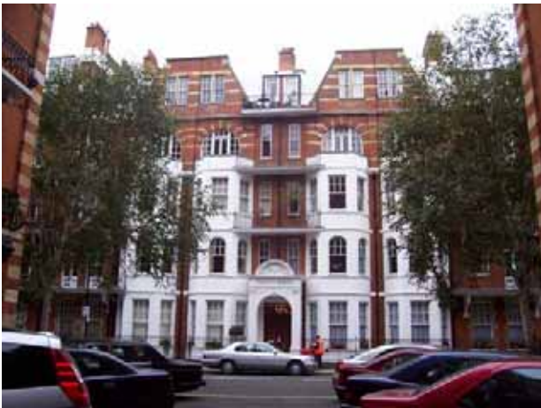
Figure 49: No.160-169 Ashley Gardens, Emery Hill Street
