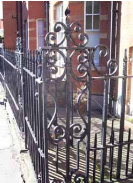
Figure 78: Early 20th century railings with wrought iron twisted leaves on corner of Emery Hill Street
