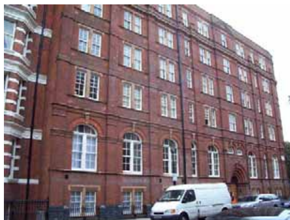
Figure 42: United House, Ambrosden Avenue
