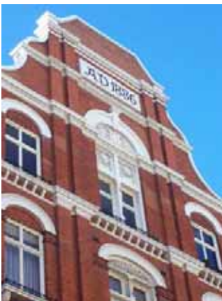
Figure 28: Dutch-style gabled roof of western Carlisle Mansion blocks
