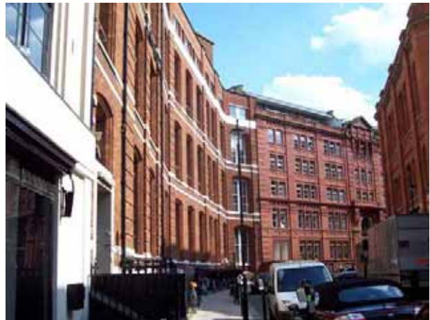
Figure 12: Victorian Warehouses in the north of the conservation area
