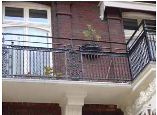
Figure 79: Balcony No.1-14 Ambrosden Avenue
