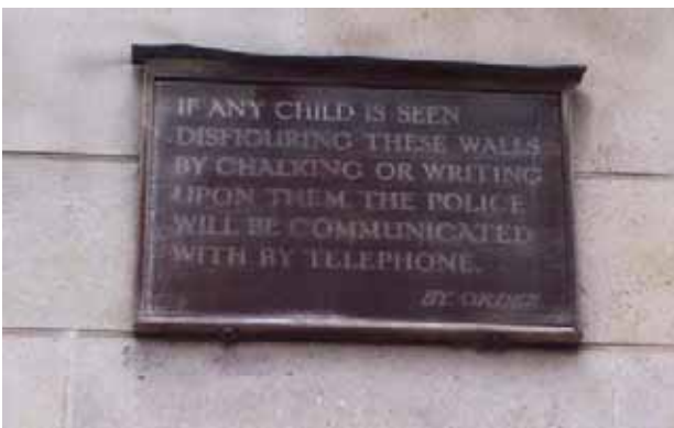
Figure 89: Wall mounted sign on Ambrosden Avenue side of Clergy House - "IF ANY CHILD IS SEEN DISFIGURING THESE WALLS BY CHALKING OR WRITING UPON THEM, THE POLICE WILL BE COMMUNICATED WITH BY TELEPHONE."
