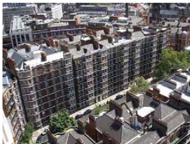
Figure 47: View of Thirleby Road from campanile
