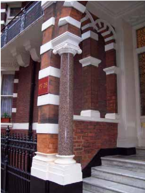
Figure 44: Nos 15-28 Ashley Gardens, Ambrosden Avenue
