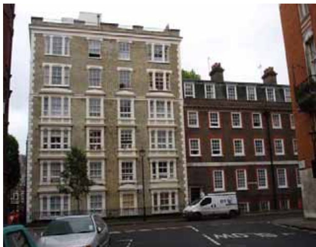
Figure 52: Improved Industrial dwellings flats and 29 Francis Street
