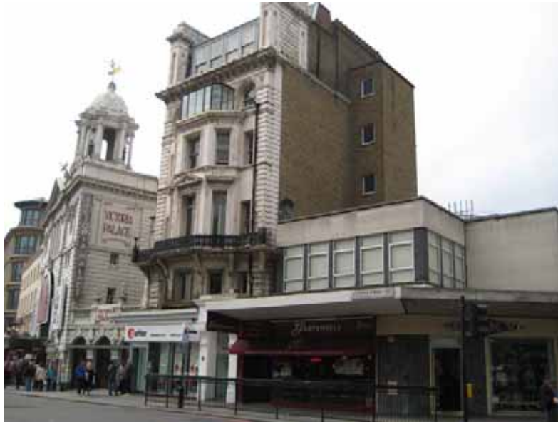
6. (l-r) Victoria Palace Theatre, Betting Shop, Garfunkles Restaurant & Risky Clothing
