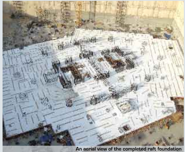
An aerial view of the completed raft foundation
