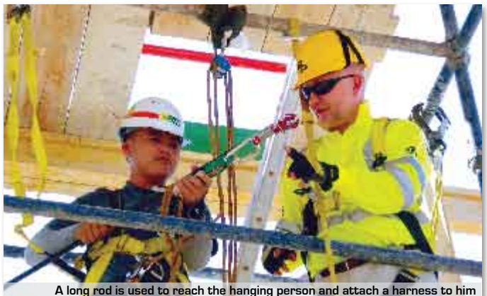
A long rod is used to reach the hanging person and attach a harness to him
