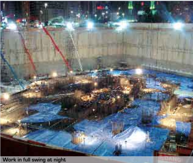
Work in full swing at night
