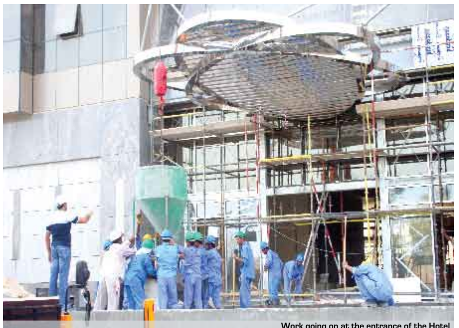
Work going on at the entrance of the Hotel
