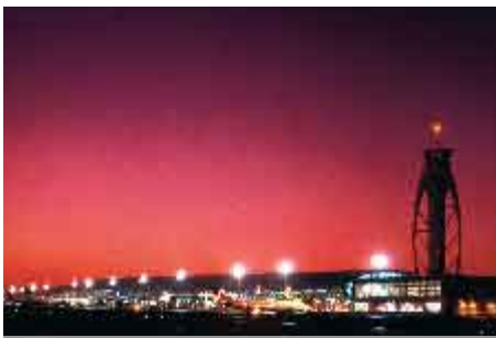
Sheikh Rashid Terminal at Dubai International Airport
