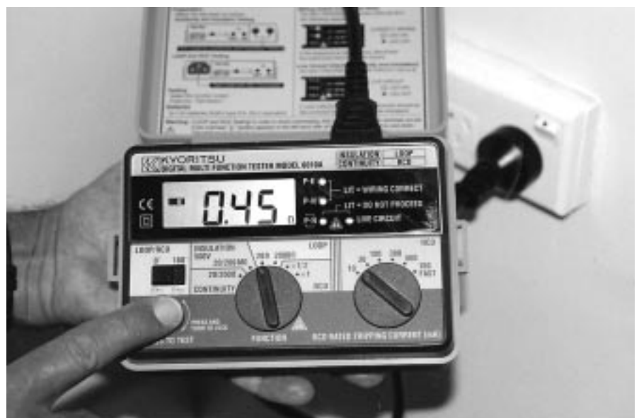
Meter being used to measure fault-loop impedance
