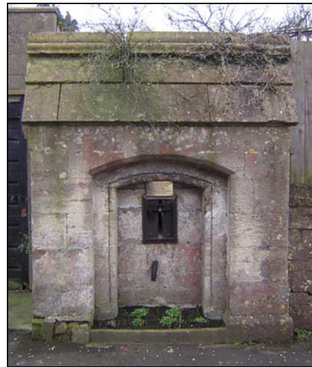
Vegetation and water damage to listed water pump
