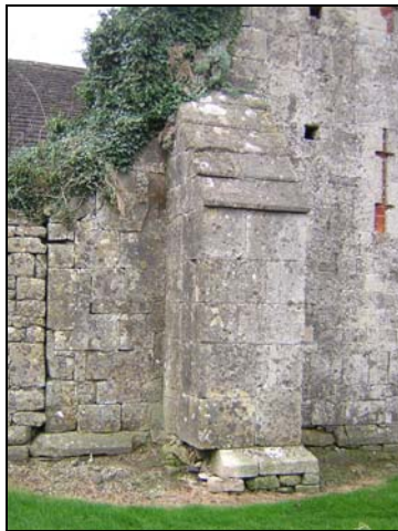
Base of pier of Abbey Barn showing signs of stone decay and erosion
