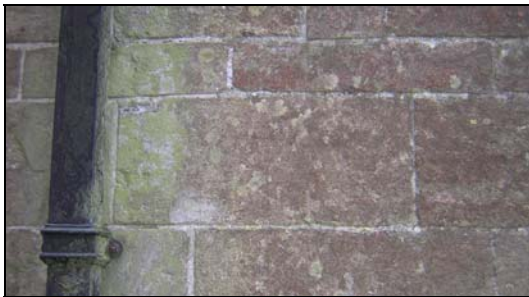
Douling stone used for dressed ashlar
