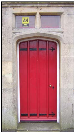
Ribbed timber plank door in dressed stone surround with fanlight
