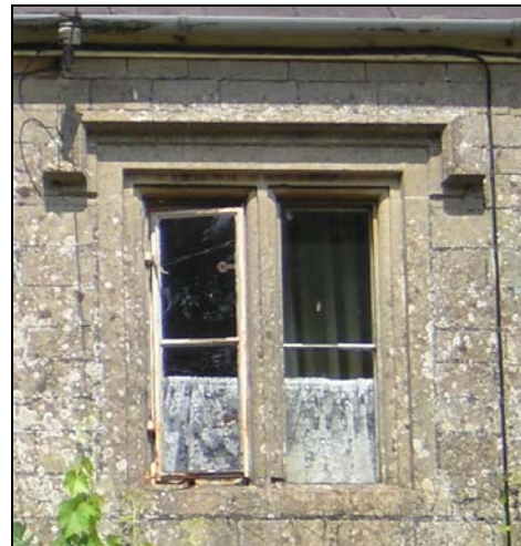
Traditional stone mullion window with iron side-hung casement and direct glazing
