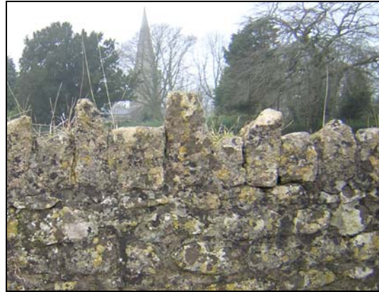
Doultong stone also used for cock and hen capping on rubble walls
