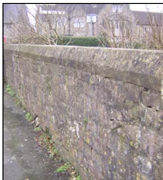
Doultong stone boundary wall with dressed stone coping
