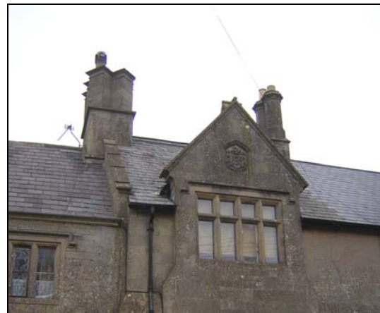
Natural Welsh slate roof enclosed in stone coped gables
