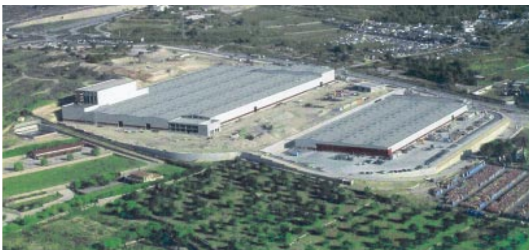
Construction work on the new Villanueva y la Geltru Telecom Cables factory in Spain has almost been completed.
