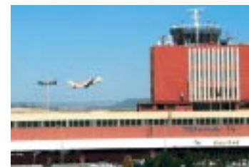
In Madrid, Pirelli Energy Cables replaced the Barajas Airport's aerial lines with underground cables.
