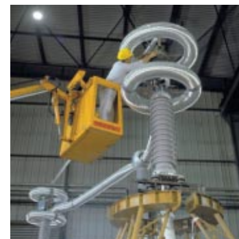
Testing high voltage energy cables.
