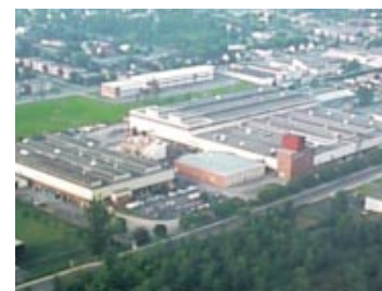
The Saint Jean plant in Canada was expanded by Pirelli Energy Cables and Systems in 2003.
