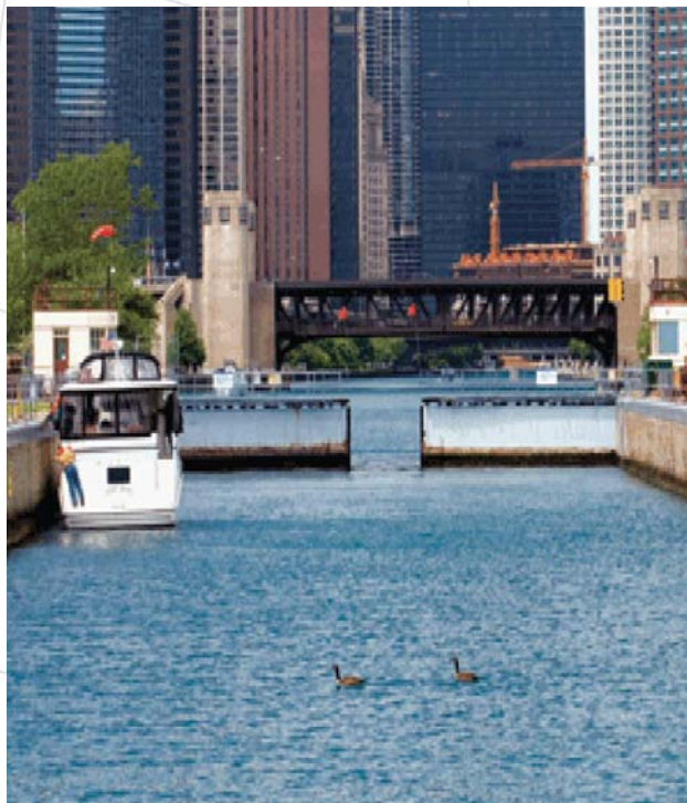
Locks are critical infrastructure in the Great Lakes system. (Left) the Chicago Lock in Chicago, Ill.
