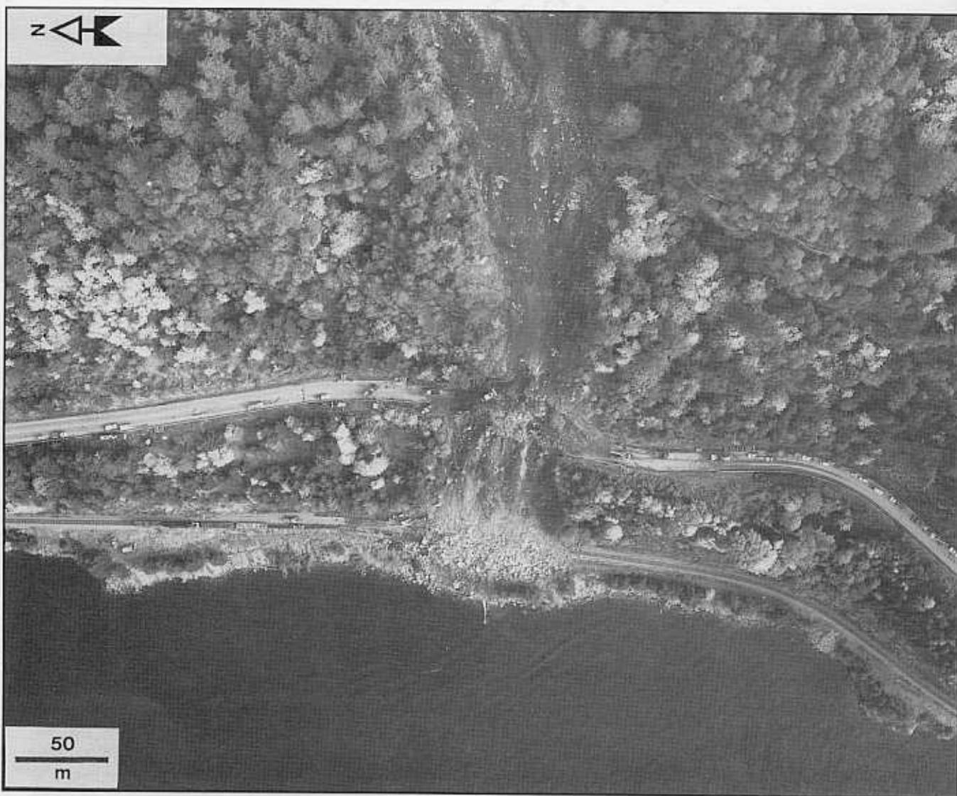
Figure 2. Aerial photograph of rockfall which covered the Sea-to-Sky Highway and B.C. Rail tracks, 4 km north of Lions Bay, October 1990 (Photo courtesy of Selkirk Remote Sensing, Richmond, British Columbia; negative number SRS 4466-5).
