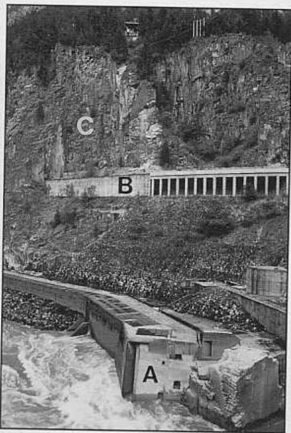
Figure 7. View of Hell's Gate fishways, A) looking upstream from the west bank of the Fraser River in 1985. Note Canadian National Railway rockfall protection structure, B) and steep jointed rock slope of Fraser Canyon wall above C) source of 1914 rockfall. GSC 1994-709B
