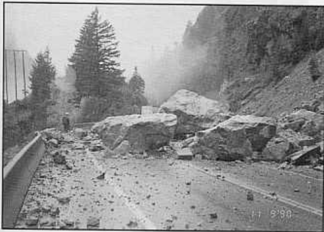
Figure 4. Rockfall on Trans-Canada Highway, Fraser Canyon, near Yale (courtesy of D. Wyllie).
