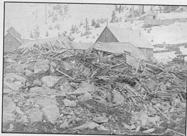
Figure 9. Destroyed buildings and rock debris at Jane Camp, Britannia mine, following the 1915 rock avalanche which resulted in 56 deaths. The Jane Camp tragedy is Canada's second largest landslide disaster, after the 1903 Frank Slide (photo by British Columbia Museum of Mining).
