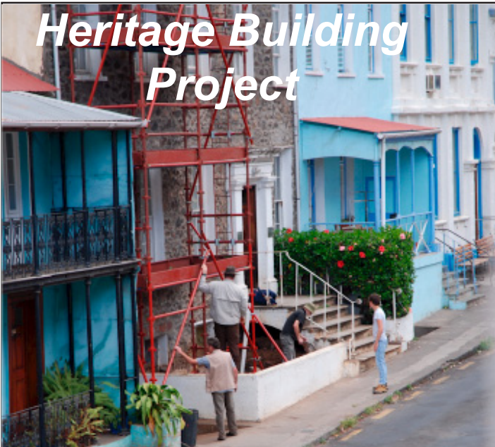
Ben Jeffs checking the scaffolding
