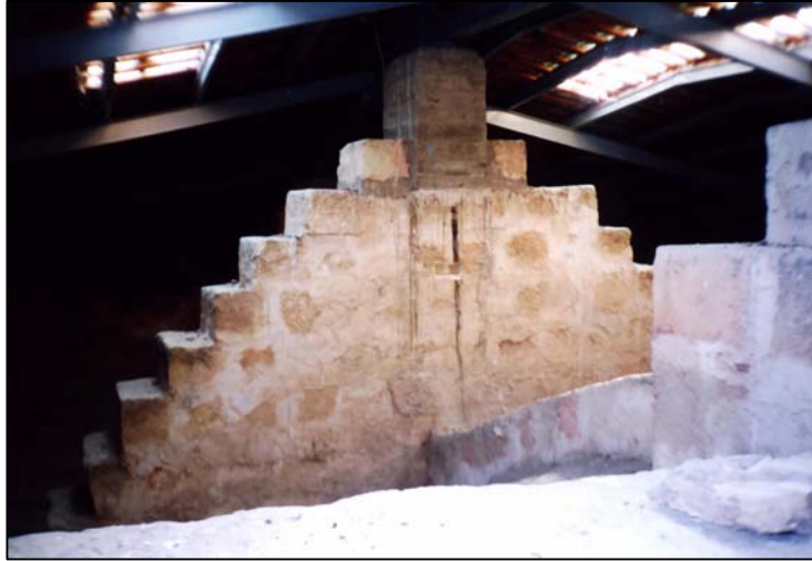
Figure 4 - Masonry Pyramid over the key of a transverse arch
