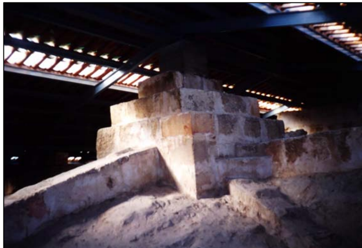
Figure 5- Masonry pyramid over the key of a vault
