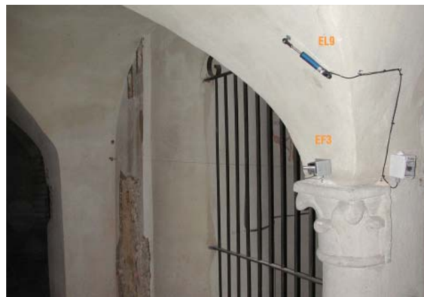
Figure 11: cable extensimeter EF3 and electric extensimeter EL9
