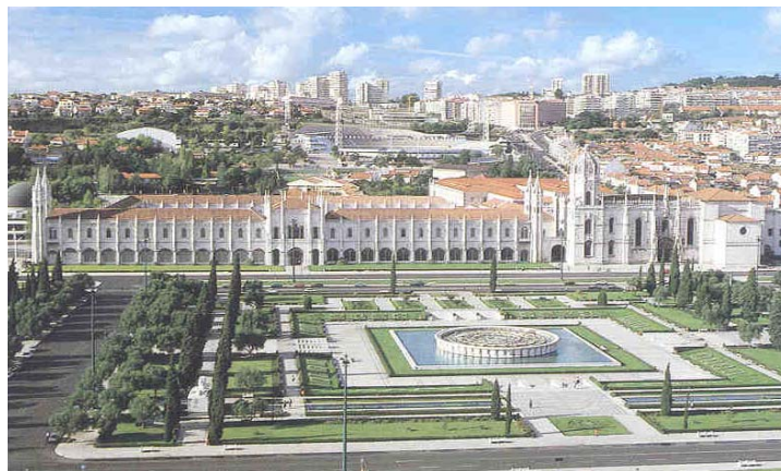
Figure 1 - General view of the Monastery of Jerónimos and the Empire Square.
