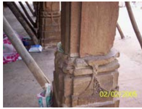
Figure A.1 – Geometry: (a) front view of Mosque (b) displaced column of mosque due to 2001 earthquake (c) repairing of periferal distress beam of tomb under progress by ASI
