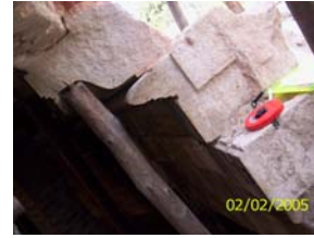
Figure A.1 – Geometry: (a) front view of Mosque (b) displaced column of mosque due to 2001 earthquake (c) repairing of periferal distress beam of tomb under progress by ASI
