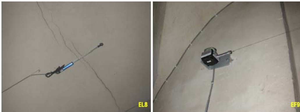
Figure 18: cable extensimeter EF9 and electric extensimeter EL8
