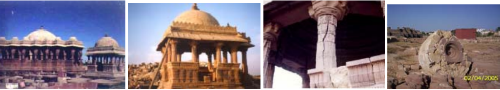
(a) (b) (c) (d) Figure A.1 – Geometry: (a) Rao Lakhaji Chhatri in Bhuj before the earthquake. The large structure on the left is the main chhatri built after the king, Rao Lakhaji, while that on the right was built after the queen. (b) Rao Lakhaji Chhatri was reduced to rubble (in the background), while the chhatri in the foreground sustained significant loosening of the masonry stones at both the sill and lintel levels. This chhatri, though still standing, is on the verge of a vertical split and complete collapse (c) Damage to stone column of the Royal Chhatri in Bhuj. (d) Close view of inner solid section of chhatri, which was damaged during 2001 earthquake.
