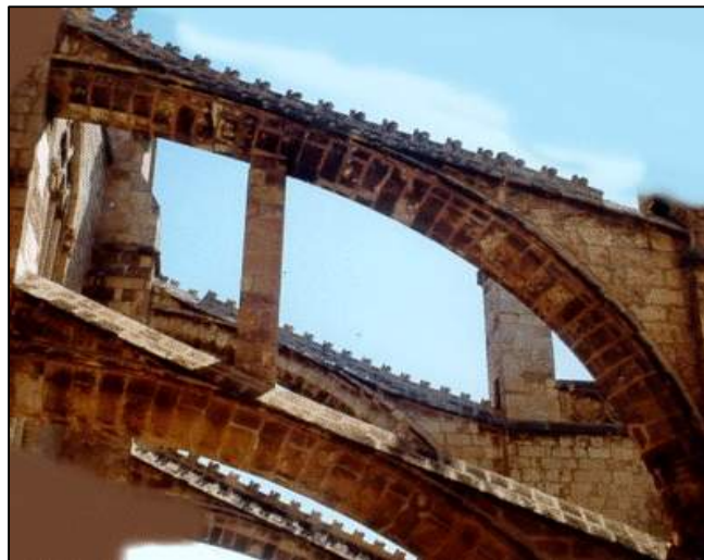
Figure 8 - Flying arch propped on a masonry pillar
