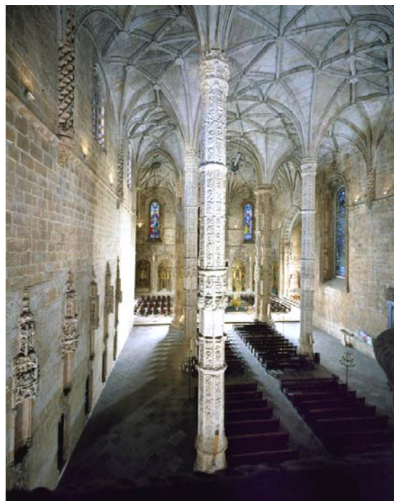
Figure 12 - "Fan vault" appearance for the church's ceilings (Source: IPPAR).
