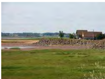
Reinforced embankments and 100m saltmarsh left to act as a natural buffer zone in the Bay of Fundy.
