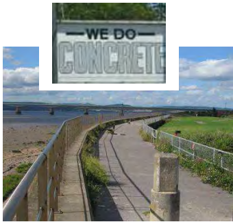
Concrete defences at high water mark along the Severn Estuary shoreline.
