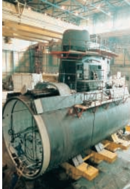
The submarine is built as a number of open, free-standing sections for exceptional ease of access.
