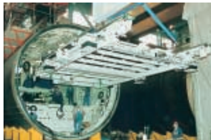
A fully assembled platform is installed in one of the sections.
