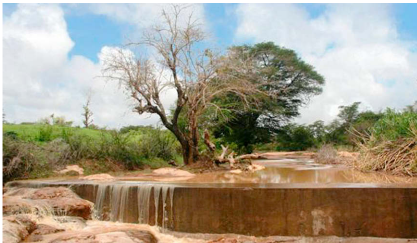
Plate 1. Example of a sand-storage dam.
