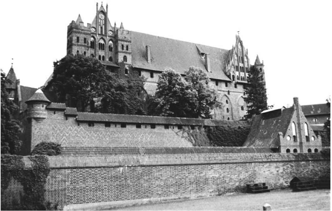
Fig. 4. Upper Castle from the Bridge Gate.
