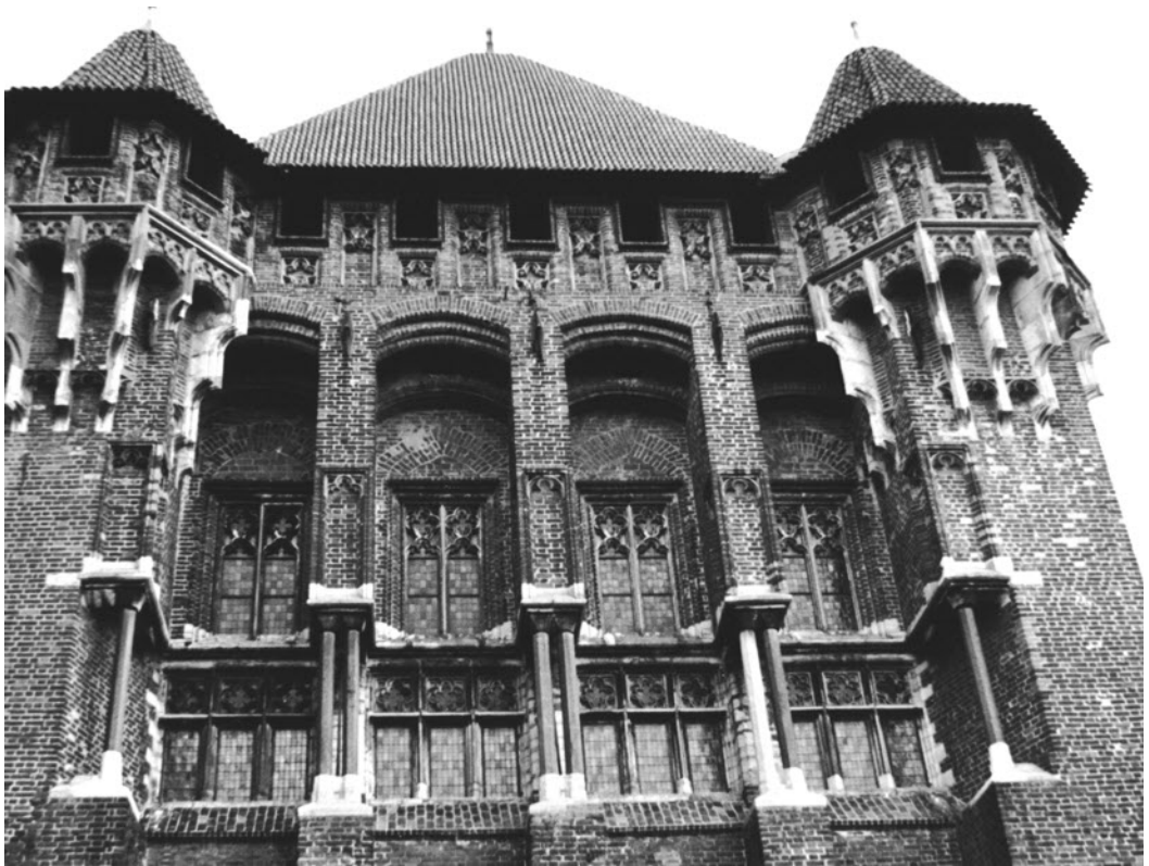
Fig. 18. Grand Master's Palace. West façade with windows of Summer refectory and crenellated parapet.
