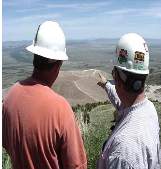
Overview of recontoured heap leach facility.
