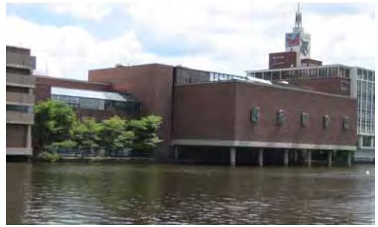
A new promenade along the face of the Museum of Science and its garage would be greatly beneficial.
