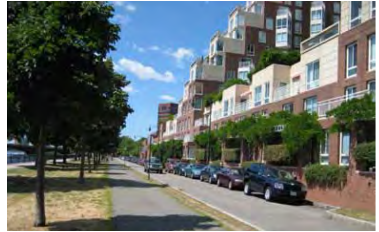
Cambridge Parkway was 80 feet wide before it was narrowed during the East Cambridge Riverfront project; it was narrowed to 20 feet to create a linear park for recreational use.
