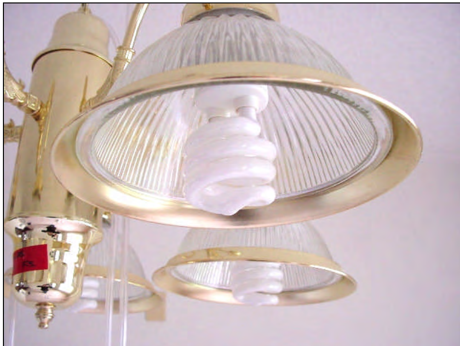
Figure 5. Compact fluorescent lamp in a Test House.
