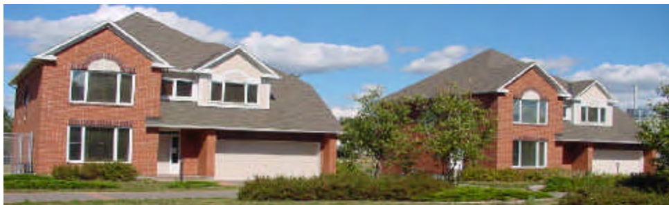
CCHT houses during the summer months.
