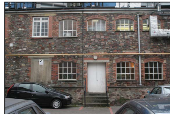
Rear kitchen extension c1952
