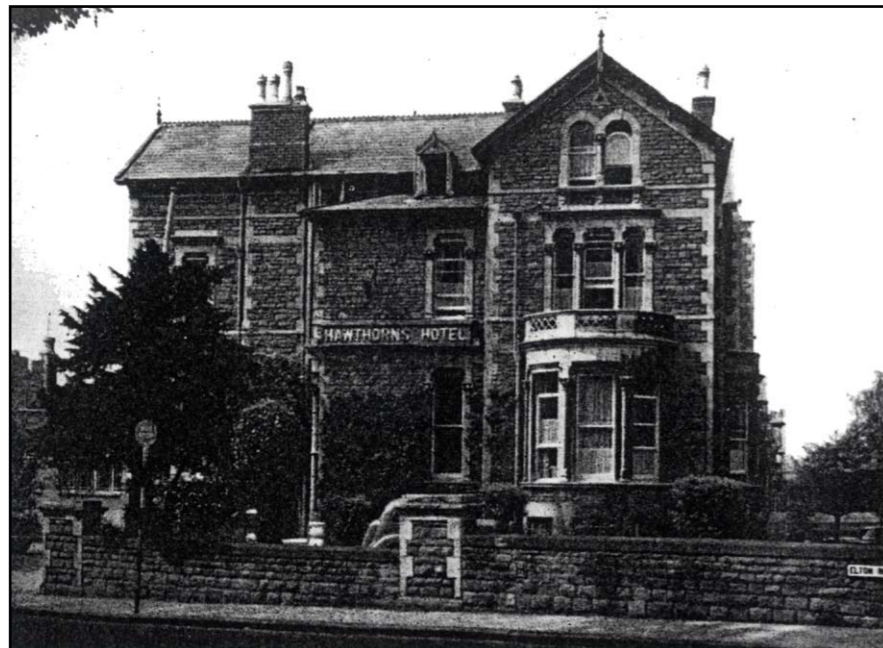
No.12 Elton Road in 1929 prior to alterations
