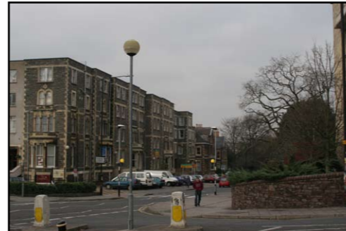
Woodland Road elevation showing confused horizontal lines, poor rhythm and general lack of quality
