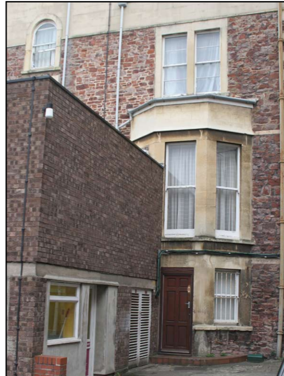
1990s brick laundry block truncates Victorian Bath stone bay window
