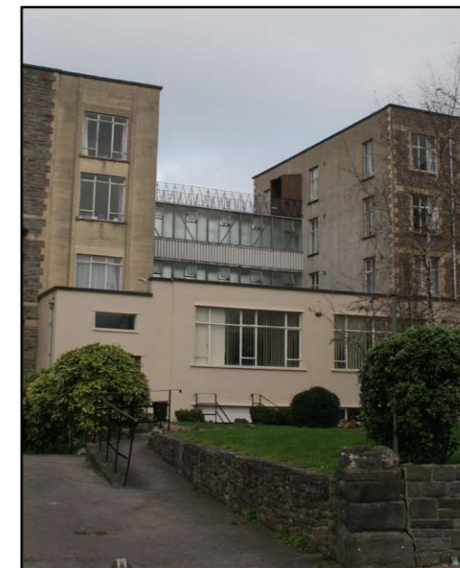
Inappropriate design detracts from original quality
