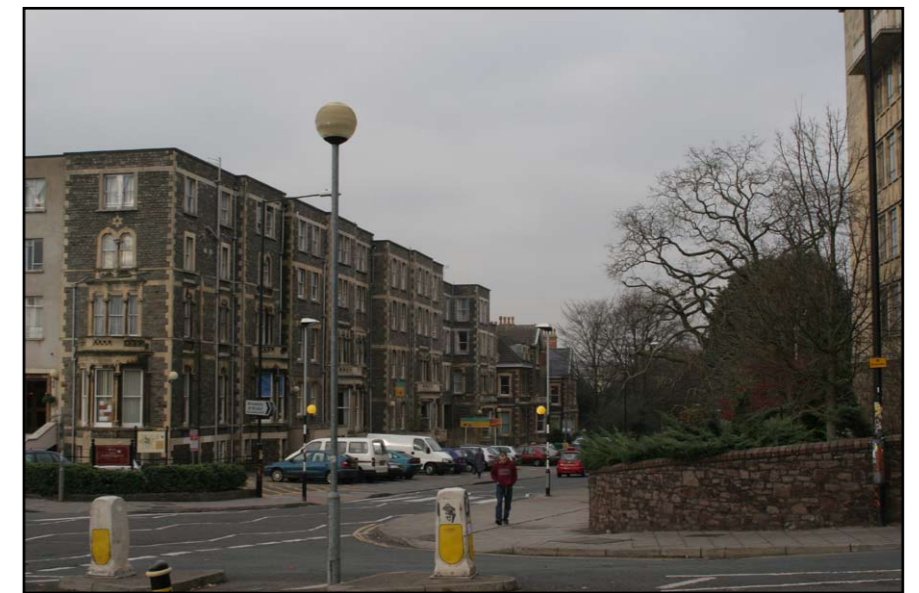
East elevation of Hawthorns (from South)
