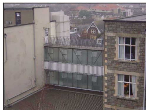
Glazed 3-storey walkway linking 2 blocks of accommodation
