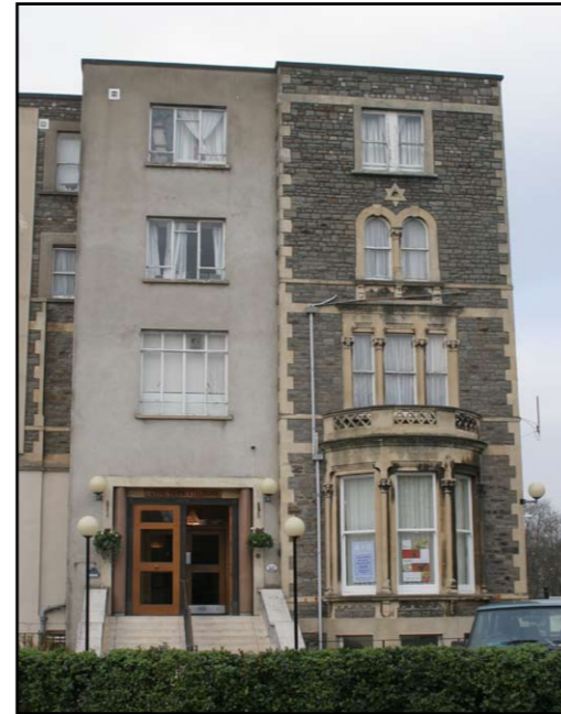
Altered roof-line and additional storeys have destroyed the original architectural movement of the villa
