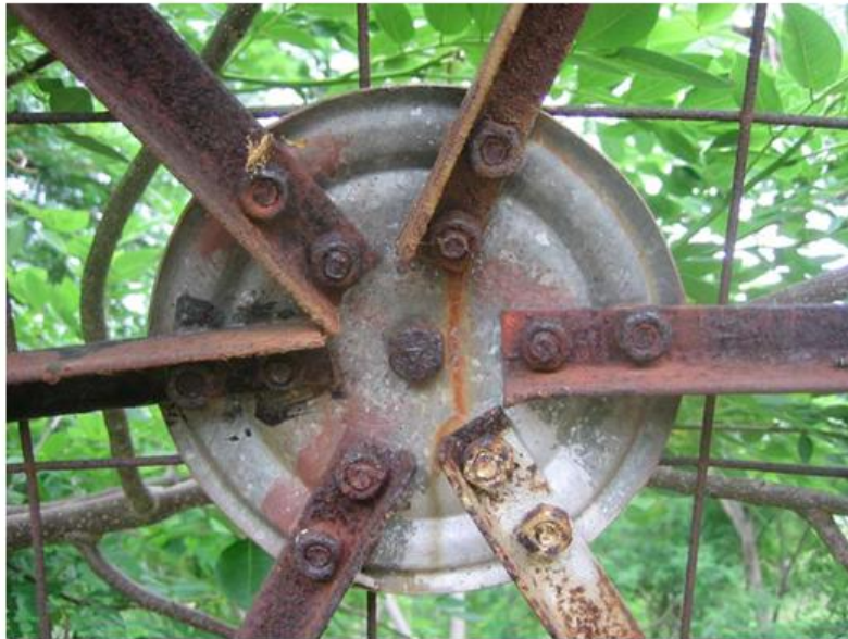
Figure 17: Close up of Pabal dome joint
