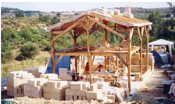
Figure 16. Ossature bois
