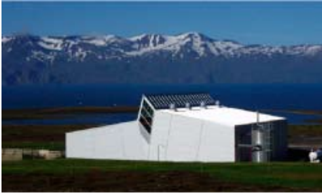
Figure 7: Husavik Kalina Binary Plant.
