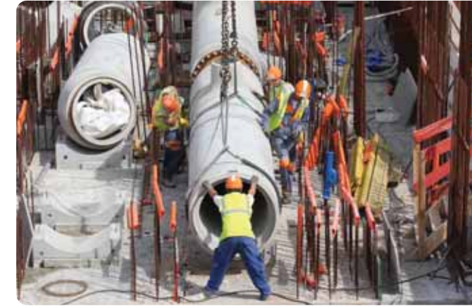
Cooling pipes being installed at EDF's new nuclear plant in Normandy
