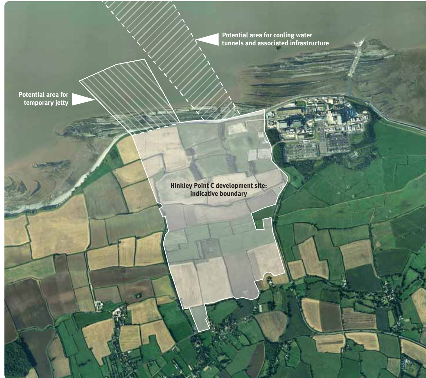
Aerial photograph of Hinkley Point
