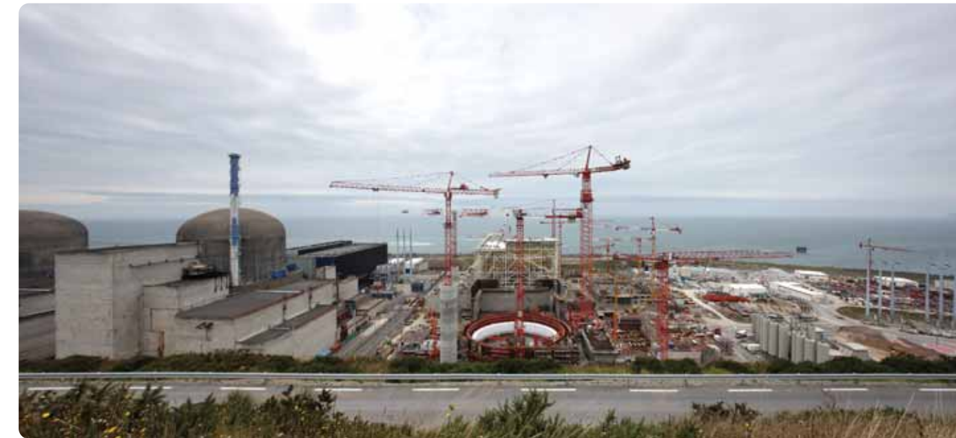
Progress at EDF nuclear power station at Flamanville, Normandy
