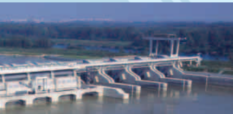
The Freudenau Power Plant on the Danube
