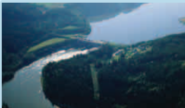
The Edling Power Plant on the Drau
