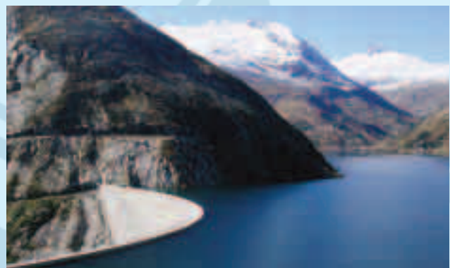
The Kölnbrein Reservoir of the Malta storage power plants
