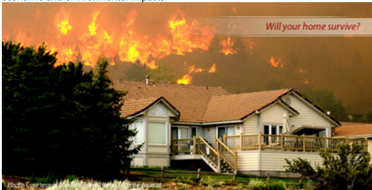
Courtesy: Living With Fire/Nevada Fire Safe Council
