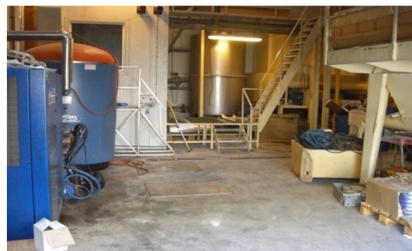
Figure 13: Room where the waste conversion was carried out 6 years ago.
