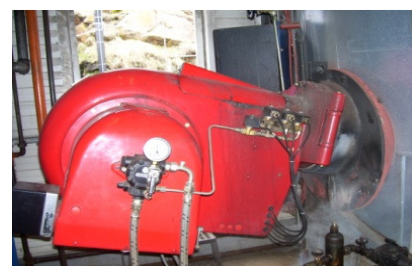
Figure 24: Compressor using in Royal Greenland Sisimiut before the boiler.
