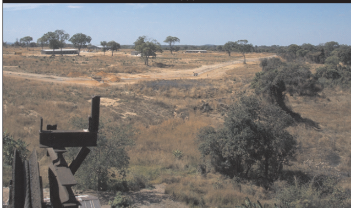
VIEW OF THE PLANNED CONCENTRATOR SITE FOR KINSEDA MINE SHOWING THE EXTENT OF BUSH CLEARING COMPLETED IN 2006
