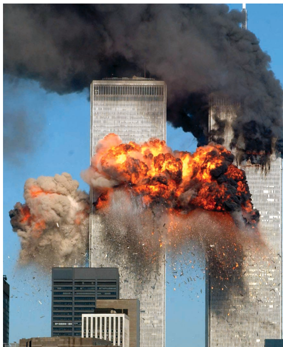
Figure 1. Flames and debris exploded from the World Trade Center south tower immediately after the airplane’s impact. The black smoke indicates a fuel-rich fire (Getty Images).
