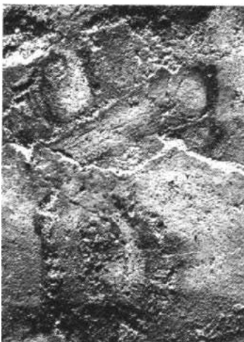
Figure 4. West wall, north bay, detail of Christ Healing the Man with the Unclean Spirit in the Synagogue at Capernaum, in raking light, showing the condition in 1979.
