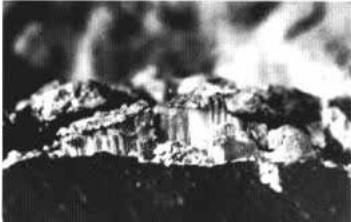
Figure 6, top. Mechanical damage due to carelessness is evident here at the level of the ledge that runs around the sarcophagus chamber (detail of Fig. 7). 1986.
