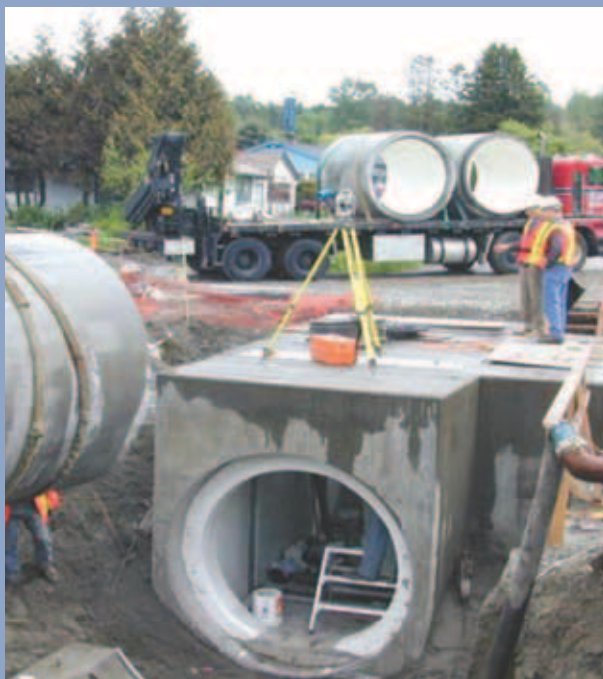
Installing Metro Vancouver trunk sewers, South Surrey.
