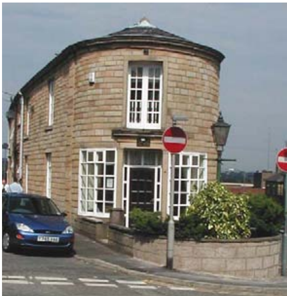
Plate 17: 'The Roundabout', eighteenth-century tollhouse at the corner of Grange Lane and Manchester Road
