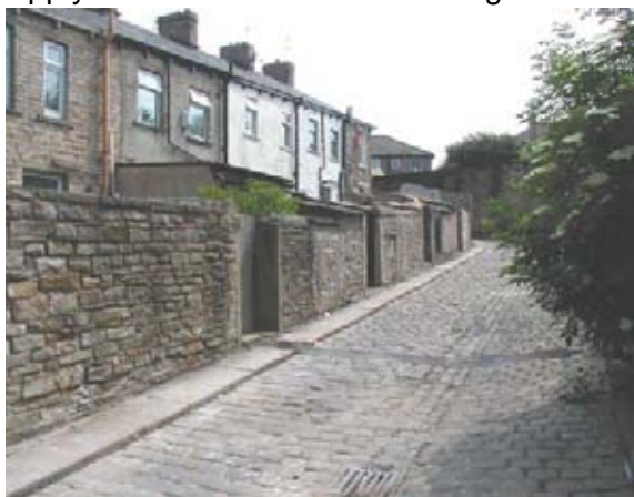
Plate 11: Scars of openings for ashpit cleaning and coal delivery, Back Adelaide Street
