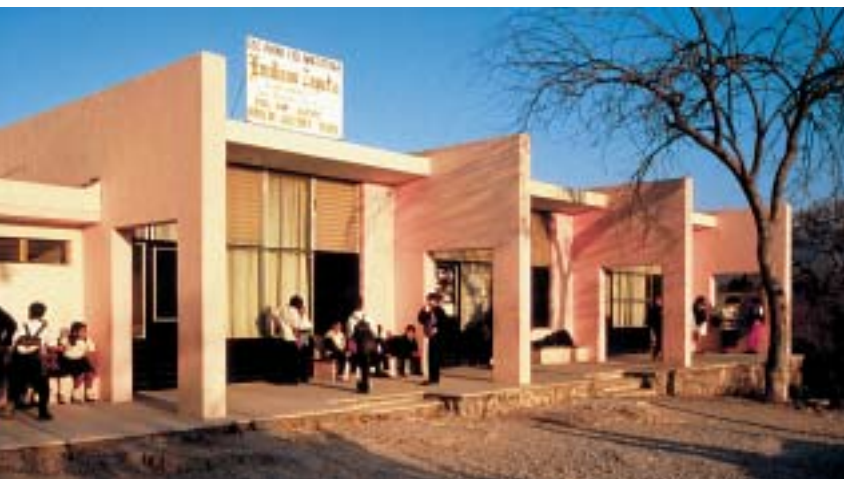
Mexico Design/Build Studio The Howard S. Wright Endowed Chair also provides support for an international design/build program run by Professor Sergio Palleroni in cooperation with Badanes. The studio has completed numerous projects in Mexico, including this school (left) and clinic (right).
