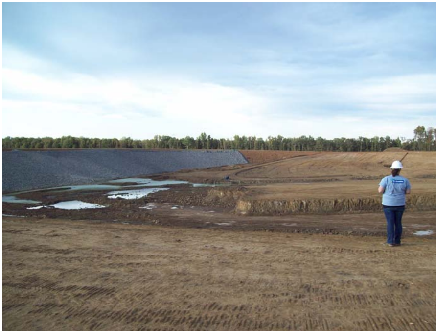
Little Red River Reservoir near Searcy, AR during Construction
