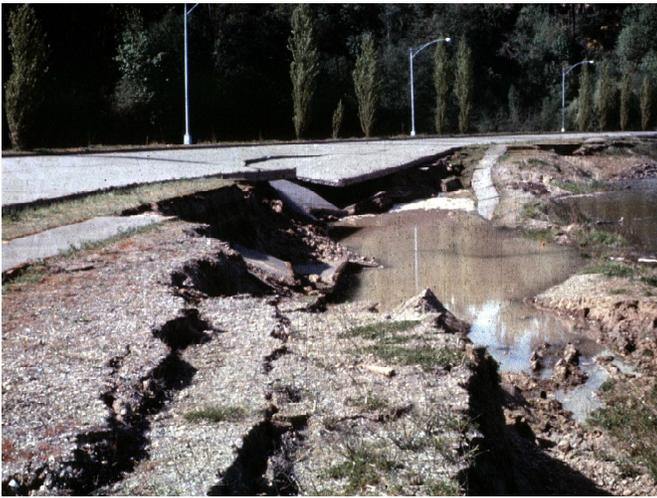
**Liquefaction can destroy roads, as the 2001 Nisqually, Washington earthquake did to this street outside Olympia. Many stretches of Highway 101 and other coastal roads in Cascadia are vulnerable to this type of destruction. Photo: T. Walsh, Washington Division of Geology and Earth Resources**
