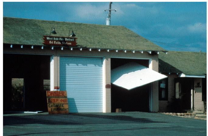
In the 1983 Coalinga, California earthquake, this fire station was badly damaged (note the skewed door). If rescue equipment can't get out of the station, it can't be used when needed after an earthquake. Photo: M.G. Hopper, USGS
