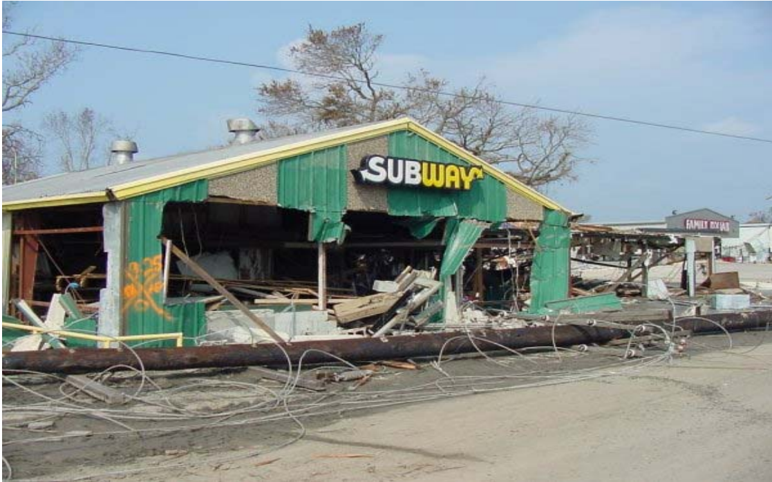
Picture 1. Example of damage in Cameron, LA caused by Hurricane Rita. Photo taken by WFO Lake Charles, LA.
