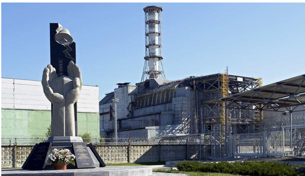
Chernobyl Nuclear Power Plant 2007
