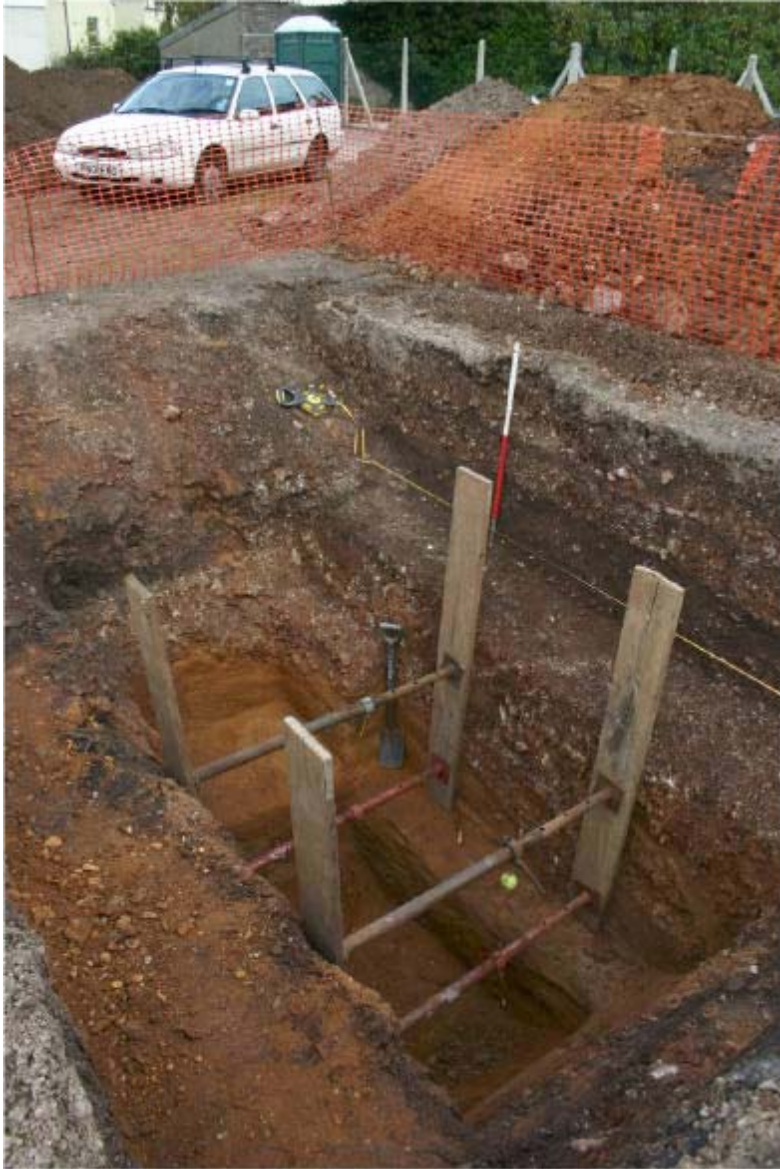
Plate 7. Excavations at Twyford House, Shirehampton into Terrace 2 deposits. Note shoring methods and access to sequence at base of trench.
