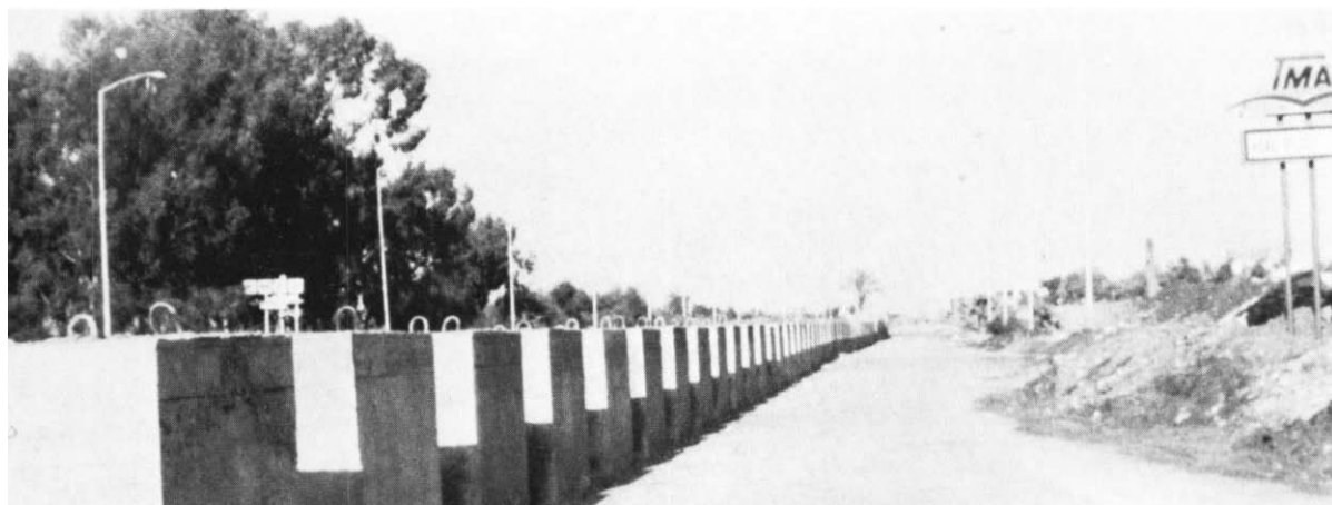
Shown in this photograph is one part of the Dragon's Teeth perimeter surrounding the 22d MAU's positions at Beirut International Airport. Nearly 800 were emplaced.
