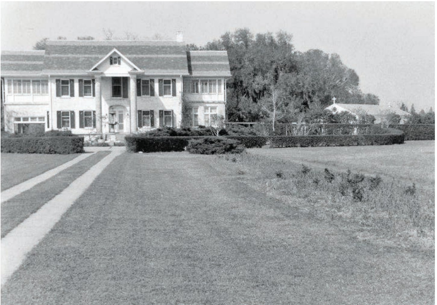
The Scanlon family's old summer home served as temporary housing for the newly arrived Cenacle sisters. They built the small chapel seen in the back ground for women who came for days of prayer.
