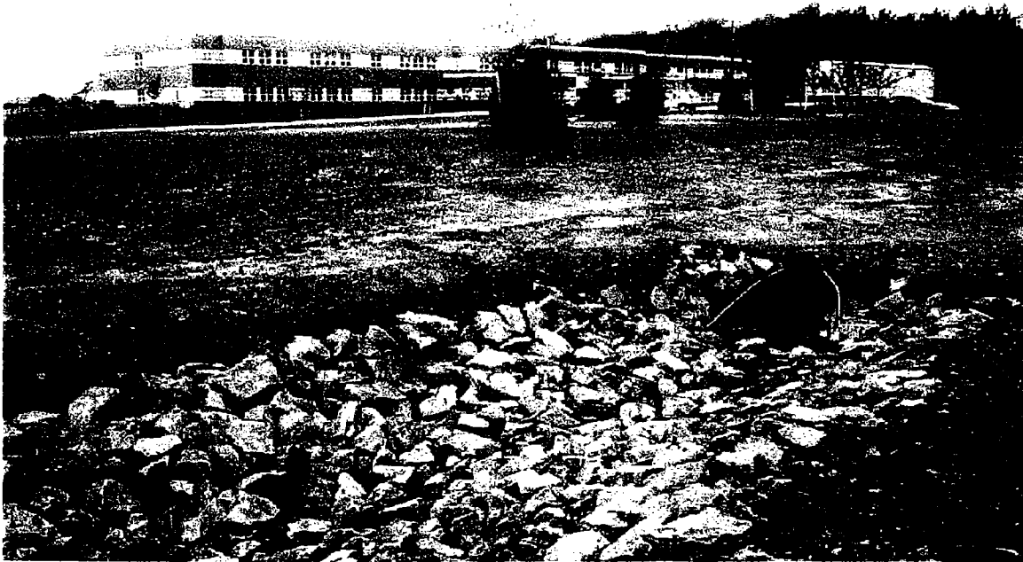
Figure 31. Storm water discharges are another symptom of development. This discharge from the newly constructed Drums Elementary School picks up great amounts of sediment and flows into the Little Nescopeck Creek.
